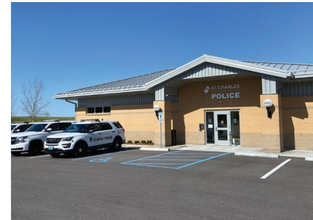
SCC's Department of Public Safety building, completed November 2021.
